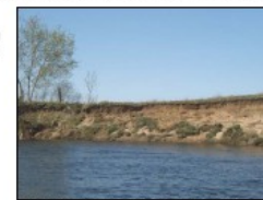
Example of erosion along the Rum River identified during a spring 2010 field survey.
