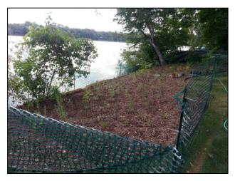
**Example project** – The photo on the left shows a lakeshore restoration on Golden Lake in Circle Pines completed in the summer of 2013. ACD provided technical/design assistance and construction oversight. The project consisted of bioengineering techniques to stabilize an actively eroding shoreline. Furthermore, native plant species were used to provide wildlife habitat. Cost-share funds were provided to the homeowner from the RCWD cost-share program.
