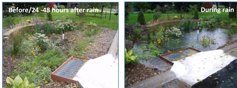
Figure 4: Rain garden before/after and during a rainfall event
