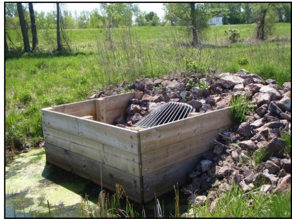
Existing outlet (left) and example of weir structure to raise outlet elevation (right)
