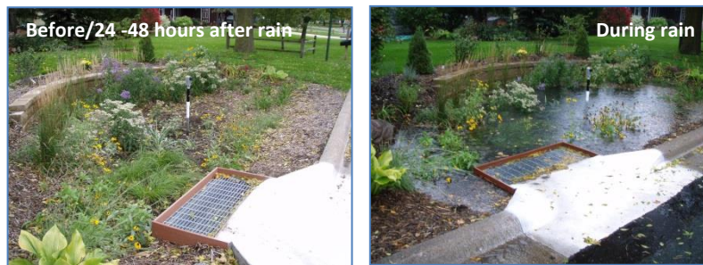
Figure 8: Rain garden before/after and during a rainfall event
