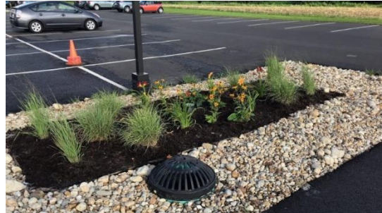
Figure 9: An HPMBS basin installed at a parking lot catch basin. The total footprint of the practice basin is about the size of one parking space.
