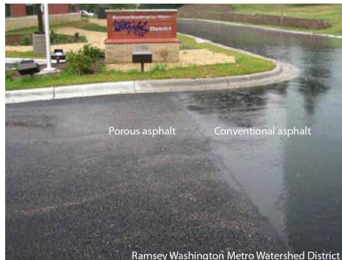
Figure 10: Photo comparing conventional and permeable asphalt
