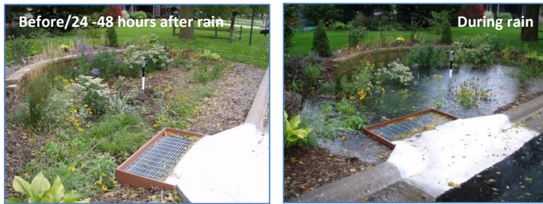
Figure 4: Rain gardens before and during rainfall events
