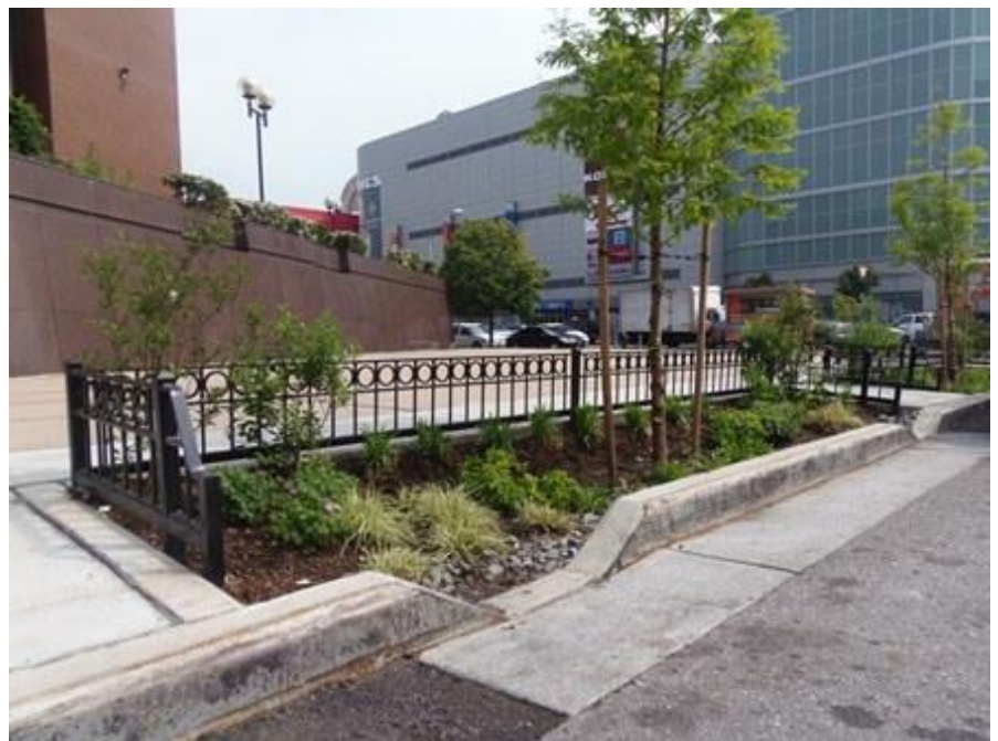
Figure 5: Right-of-way bioswale installed in New York City (NYC Environmental Protection, 2013)
