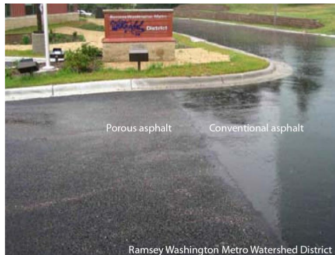
Figure 8: Photo comparing conventional and permeable asphalt
