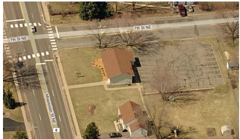
Fridley Church site prior to rain garden installation.
