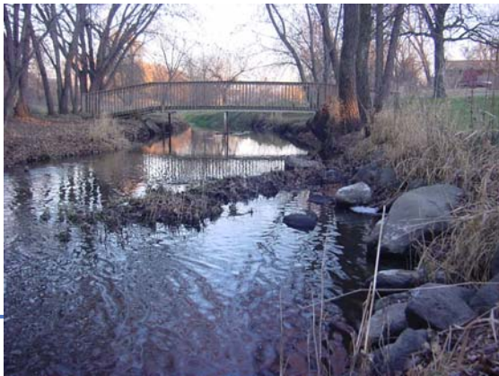
High, fast flows and removal of deep-rooted vegetation along the banks have begun eroding the banks (November 2002)
