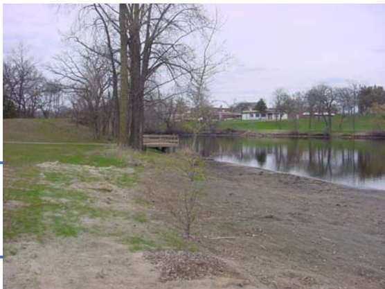
Rum River restoration site prior to buffer installation (May 2002)
