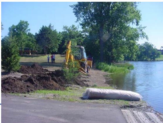
A swale is excavated to catch runoff from the boat ramp and parking lot (June 2002)
