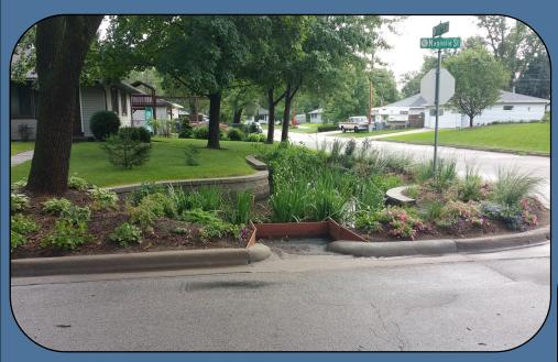
A rain garden is a constructed shallow depression that captures stormwater runoff from the surrounding area and allows the stormwater to slowly infiltrate into the soil. Rain gardens reduce runoff volumes and filter pollutants.
