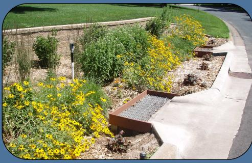
For a curb-cut rain garden, a break is created in the curb to allow stormwater runoff from the street to enter the rain garden.
