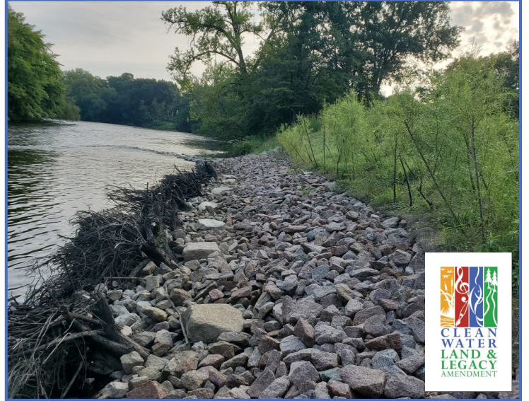
Photo nine months post-construction showing bendway weir directing flow off the previously eroded bank and native vegetation taking hold above the rock.
