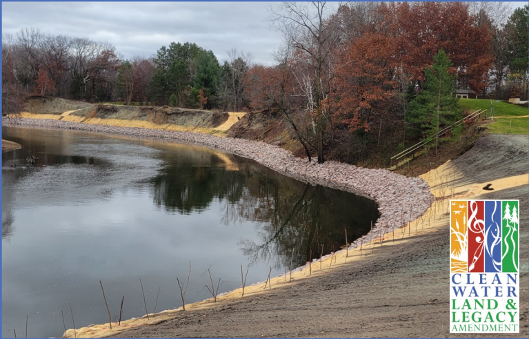
Post-construction November, 2024. Photo faces upstream.
