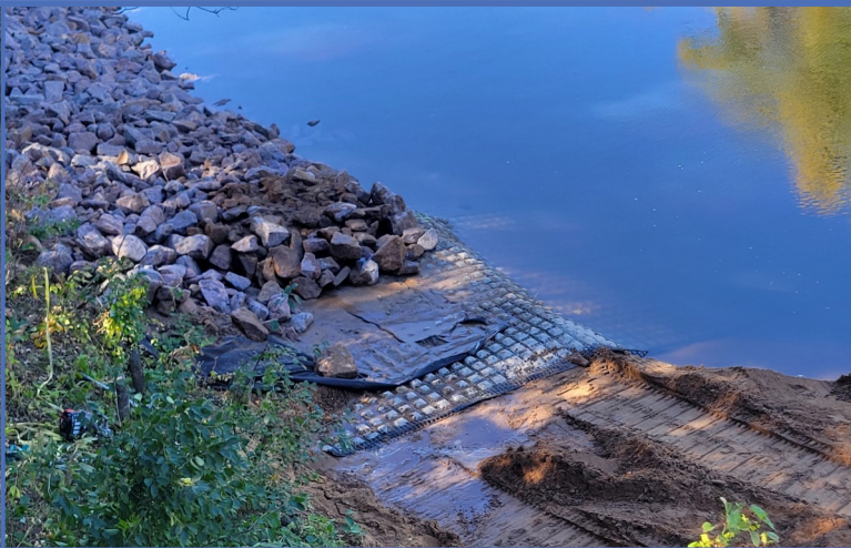
Articulated concrete block mat was launched from a low bench on the upstream 405-feet to armor the deep toe. Rock was placed above and downstream to hide the mat and armor the remainder. Banks were graded where possible, seeded, hydro-mulched, and live-staked.
