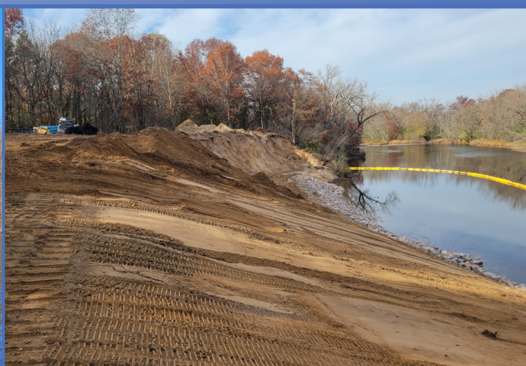
Rock riprap was used to armor the toe to a two-year flood elevation. The bank above was graded, seeded, blanketed, hydro-mulched, and live-staked to promote vegetation establishment.
