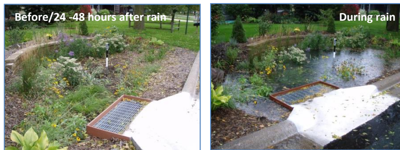
Figure 9: Rain garden before/after and during a rainfall event
